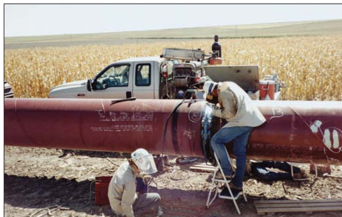
Cross-country pipe welding with Classic® 300D.
